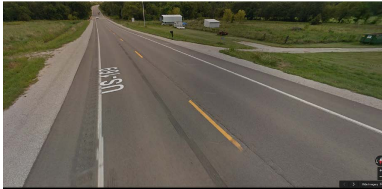
Figure 5. Rumble strip installation with gaps at driveways
